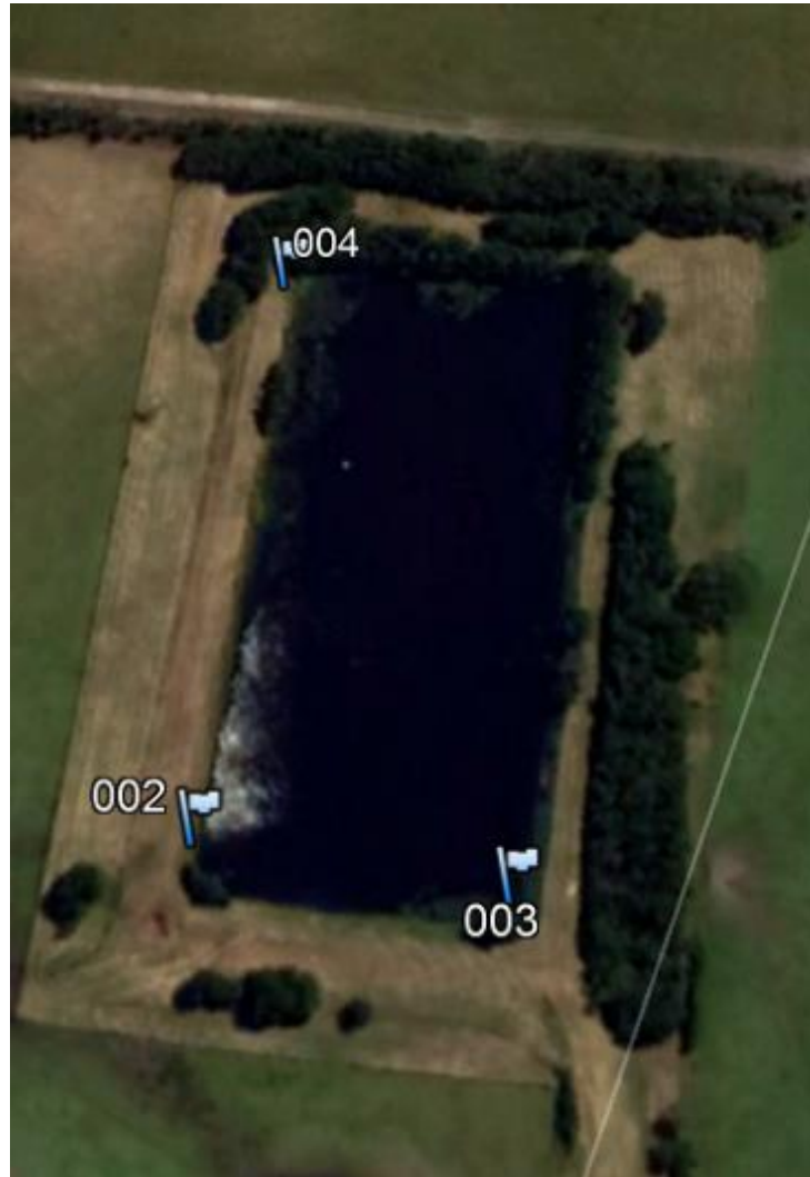
Figure 2: Walkerville Retarding Basin - Aerial view showing locations of interest
