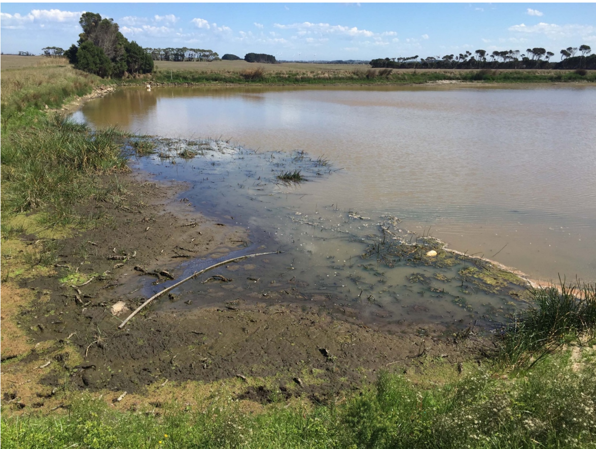
Figure 4-3: Walkerville stormwater retarding basin – 2 March 2016
