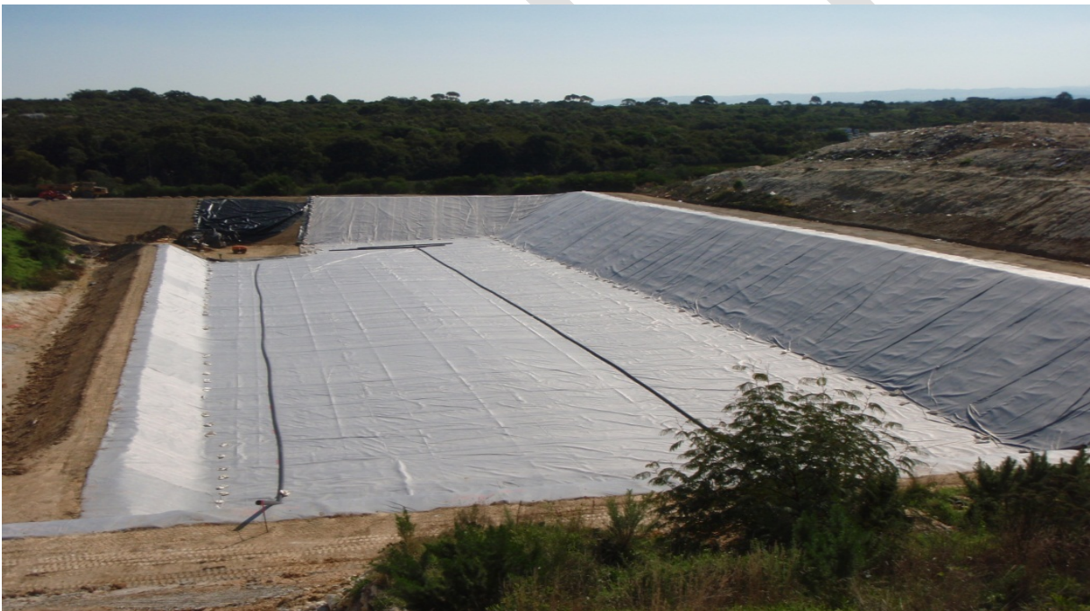
Picture 1: Koonwarra Landfill Cell 3 Construction Works
