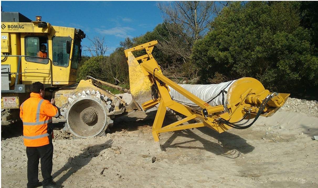
Picture 6: Tarp Landfill Cover System Installed on the Landfill Compactor
