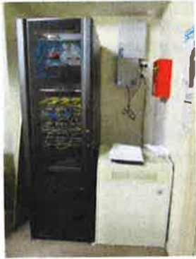
Photo: Communications Cabinet and Security Panel
