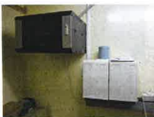
Photo: Building Occupant Warning System (Black cabinet)
