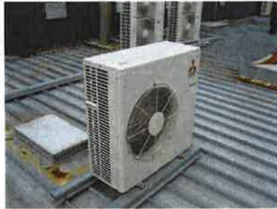
Carino's Building – Condensing unit for meeting room AC unit on roof (photo below).
