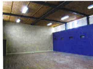
Photo: Main Hall Lighting
