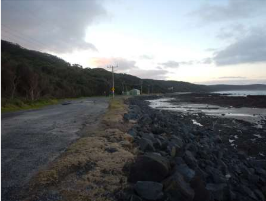
Looking north from the southern end of Bayside Drive along the existing sea wall toward the Walkerville Hall
