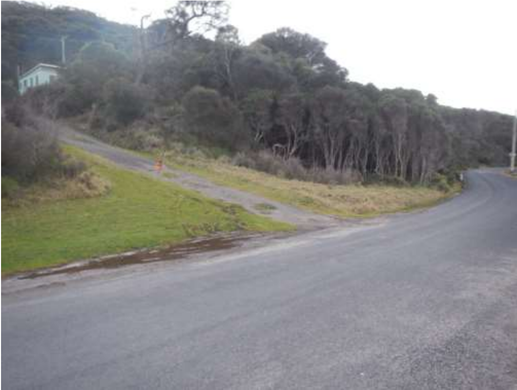
Location of proposed northern turning area looking north west. The measuring tool marks the approximate location of the 9m turning radius
