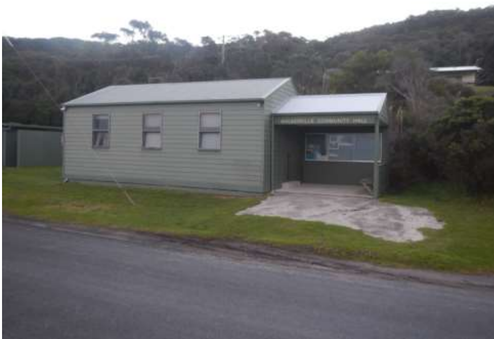
Walkerville Hall (heritage item) looking south west
