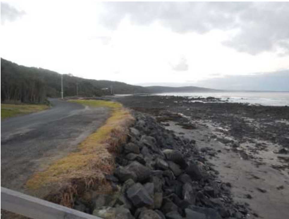
Example of erosion along the sea wall. This photo is looking north from the existing steps that go from Bayside Drive down to the beach
