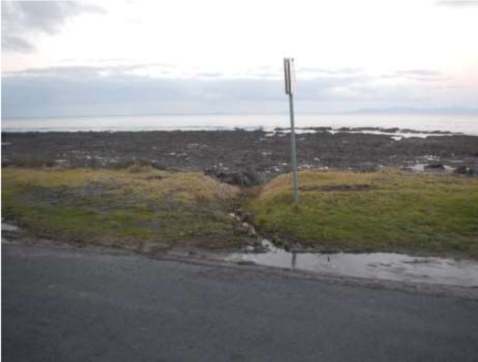
Example of existing drainage on the eastern side of the road (note pooling of water adjacent to the road)
