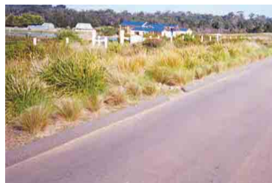
Vegetated swale conveying road runoff (Photo courtesy of Melbourne Water)
