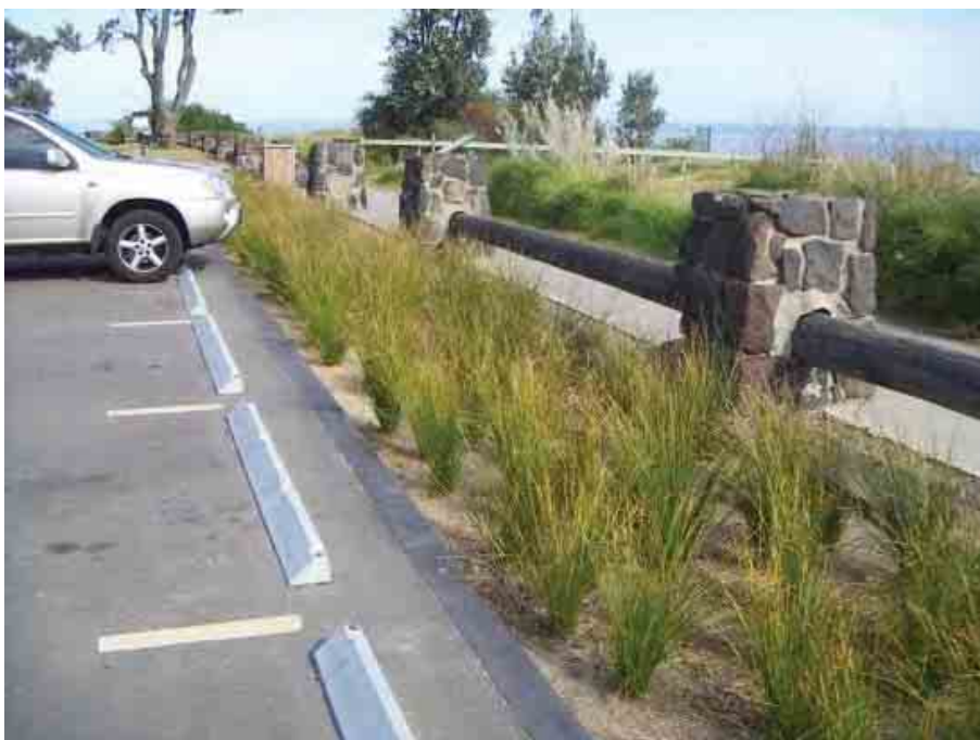
Figure 8.2 Street scale bioretention basin
