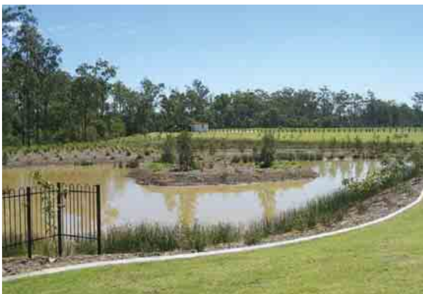
Figure 8.3 Sedimentation basin (Source: Chapter 4 Urban Stormwater: Best Practice Environmental Management Guidelines. CSIRO, 2006)
