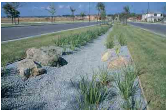
Lynbrook Estate Infiltration Trench (Photo courtesy of Melbourne Water)
