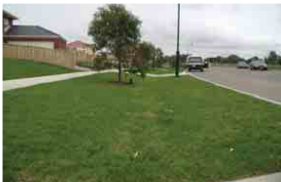
Grass swale (Photo courtesy of Melbourne Water)
