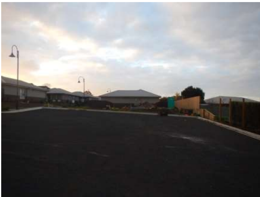
Looking north from the proposed tank and pump location.
