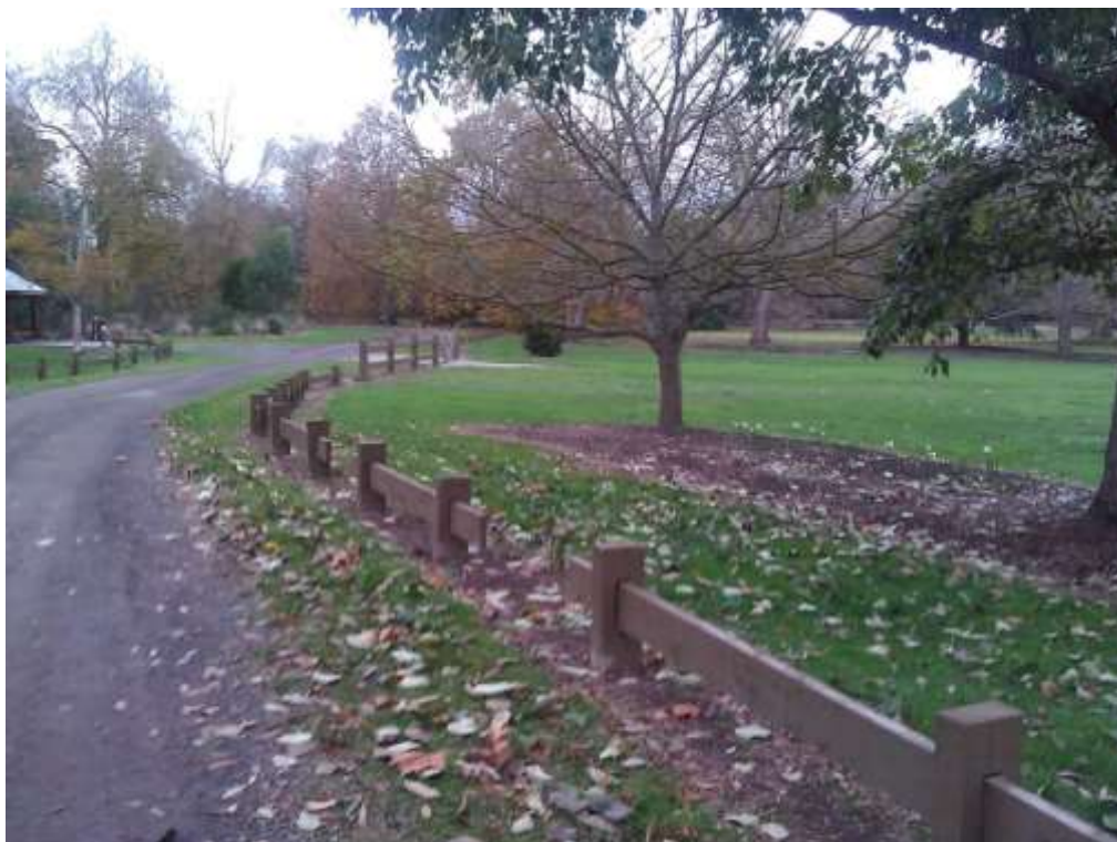
Example of post and rail fencing
