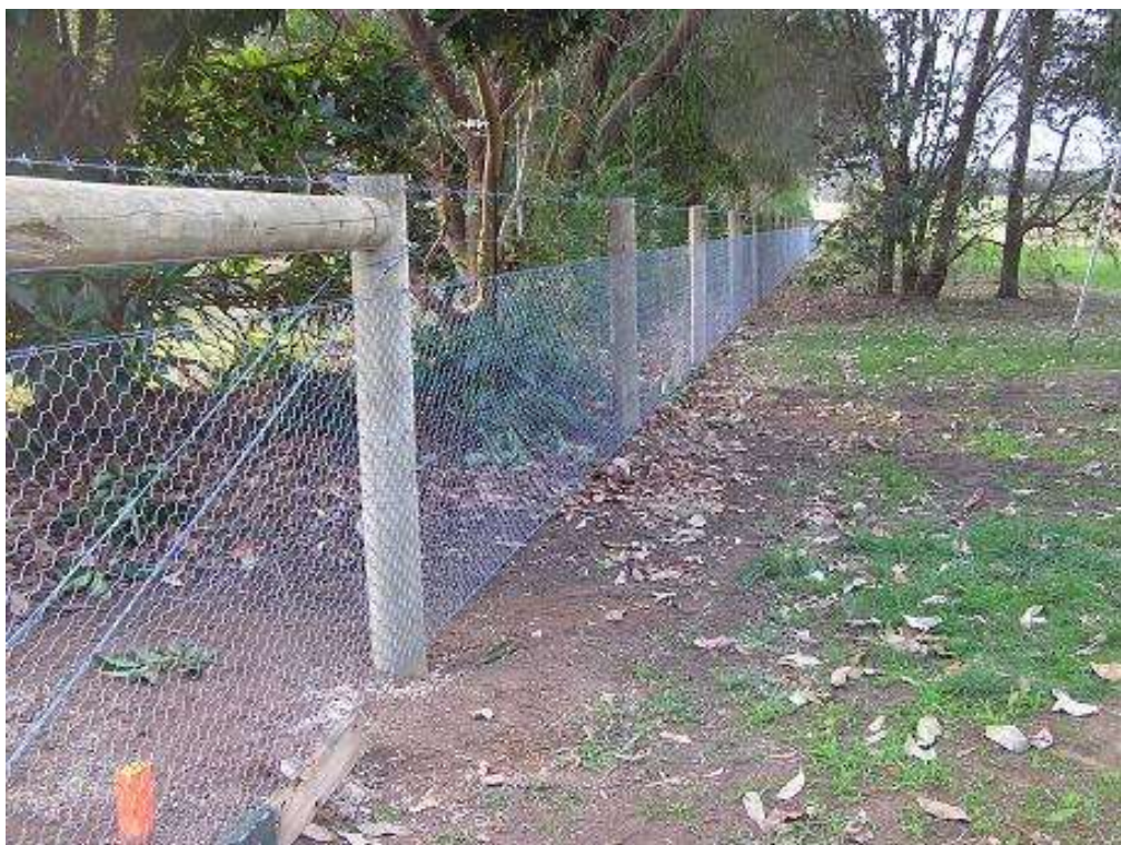
Example of fencing around river banks and revegetation zones
