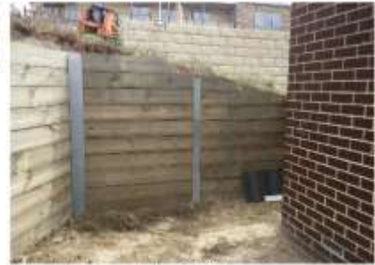
Cut and retaining wall at residential property
