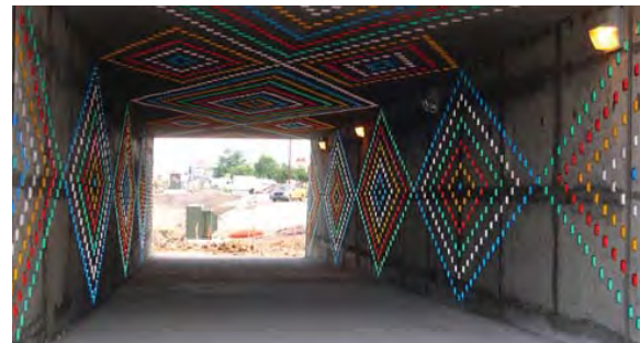
Examples of pedestrian tunnel treatments, including clockwise from top right: colourful lighting on a white surface, patterns with paint or tiles on a concrete surface or paintings and bright lighting.
