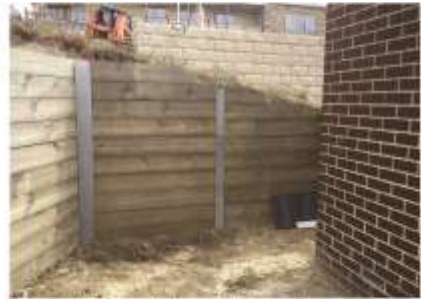
Cut and retaining wall at residential property
