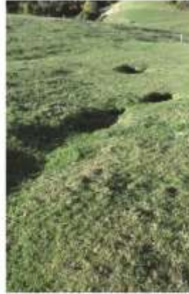
Gully erosion on rural land
