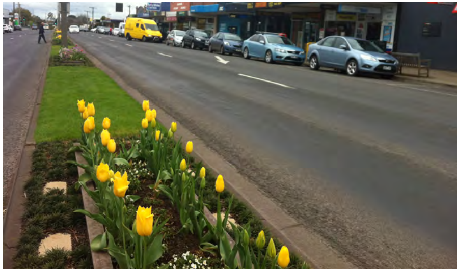
Narrow central median in Bair Street
