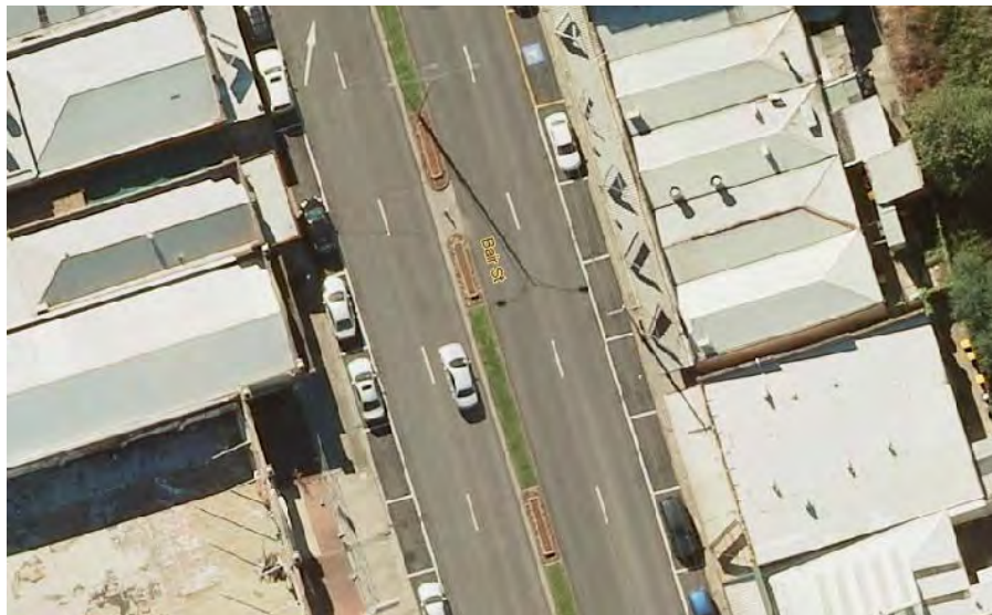
Existing two lanes on each side of Bair Street
