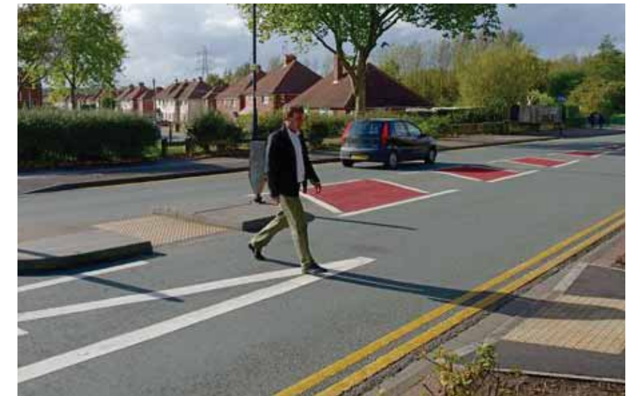
Example: Incorporate pedestrian crossing refuge area in high conflict zone, such as around the 'dog-leg'
