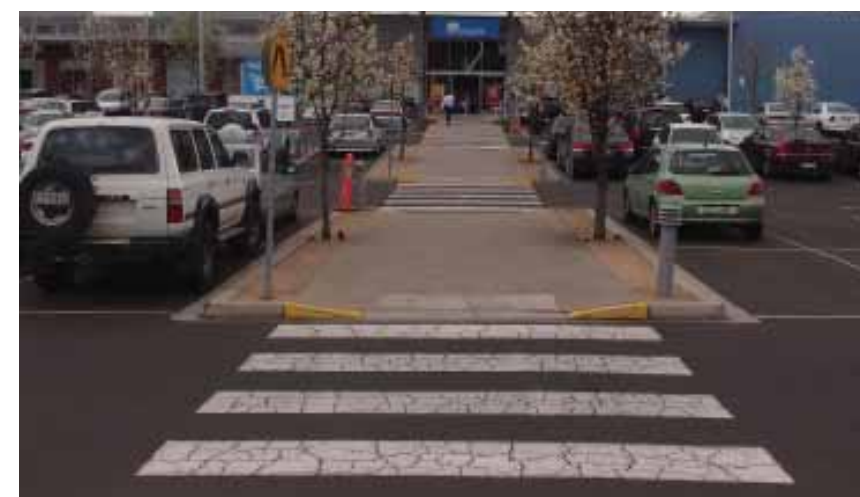
Example: central pedestrian refuge area to enable safe and comfortable pedestrian crossing
