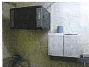
Photo: Building Occupant Warning System (Black cabinet)
