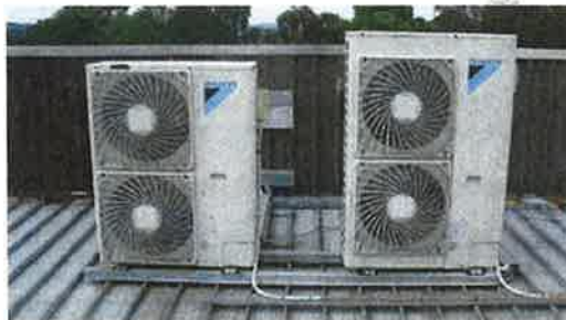
Carino's Building – Condensing unit for meeting room AC unit on roof (photo below).
