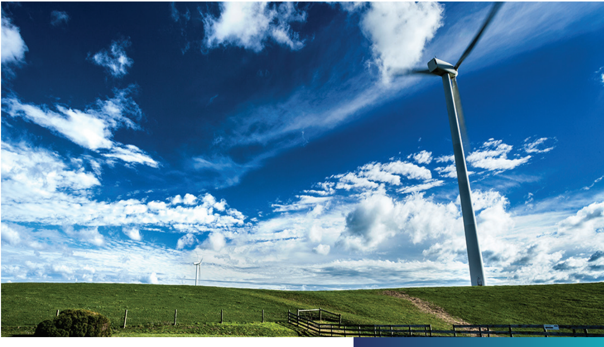
Toora Wind Turbines
