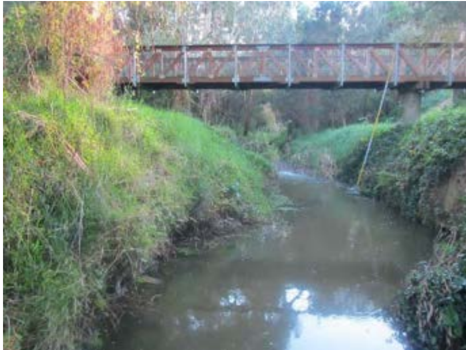
Appendix Figure A. 5 Pedestrian bridge adjacent to Scout Hall – Stockyard Creek
