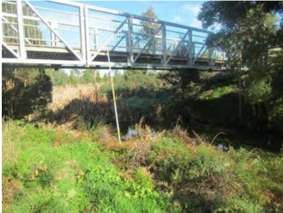
Appendix Figure B. 1 Rail Trail Bridge – Bennison Creek (1/2)
