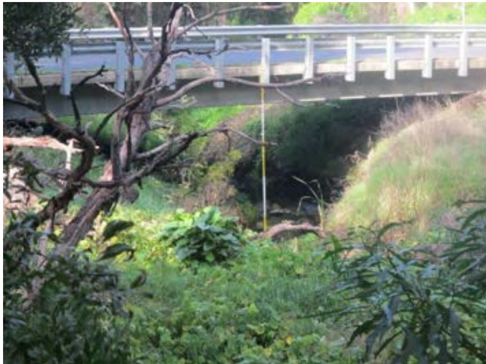
Appendix Figure A. 1 Dyrings Road Bridge 1 – Stockyard Creek (1/2)
