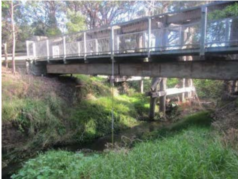
Appendix Figure B. 3 Rail Trail Bridge – Stockyard Creek (1/2)
