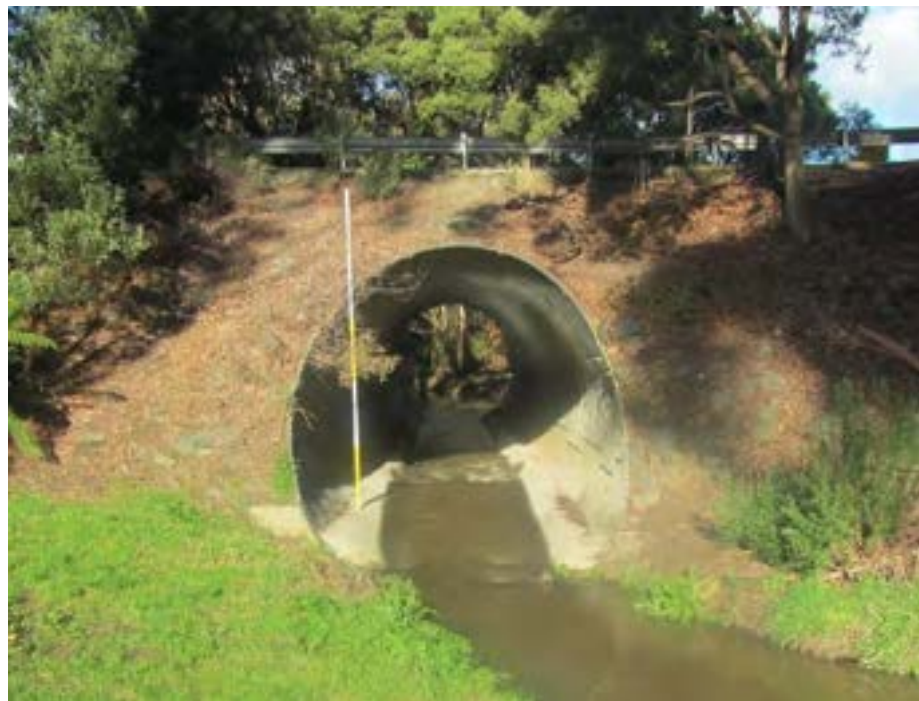
Appendix Figure A. 6 Bridge Street culvert crossing - Stockyard Creek
