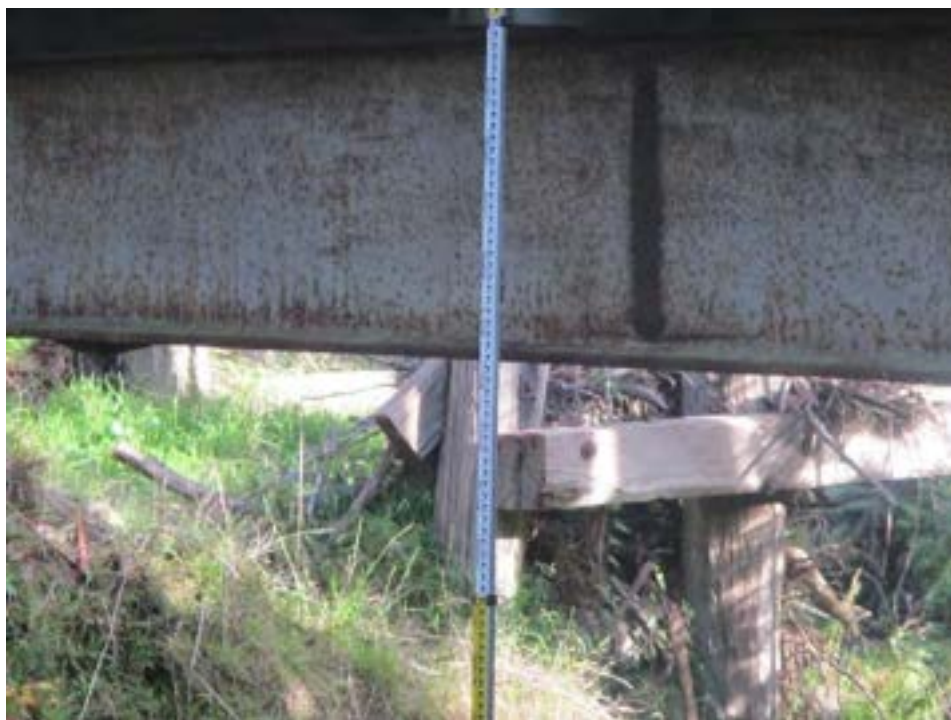
Appendix Figure B. 4 Rail Trail Bridge – Stockyard Creek (2/2)
