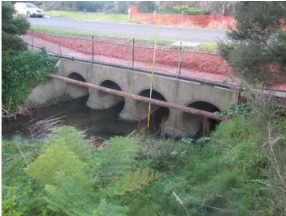
Appendix Figure A. 3 Boundary Road culverts (upstream) – Stockyard Creek
