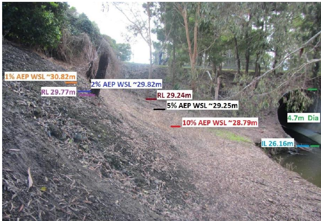
Figure 5.4 Comparison of design flood levels versus observed flood levels
