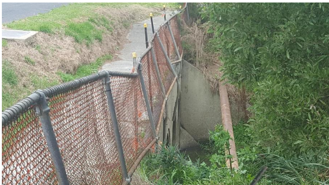
Figure 5.2 Upstream face of the Boundary Road culvert (09/04/2017)
