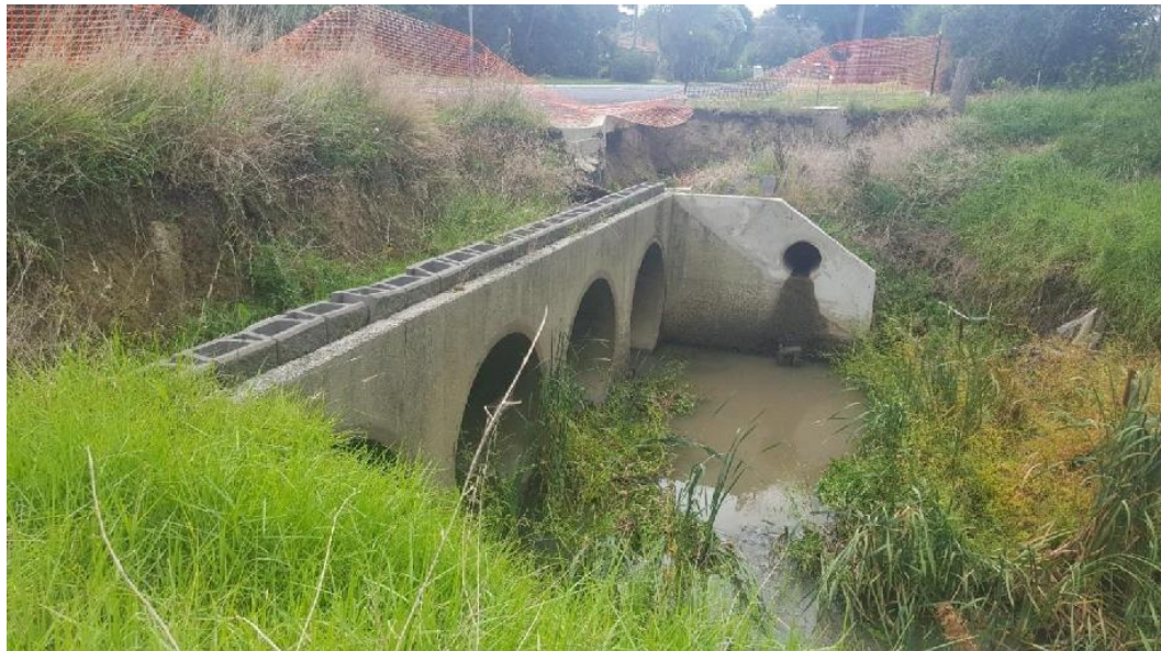
Figure 5.3 Downstream face of the Boundary Road culvert (09/04/2017)
