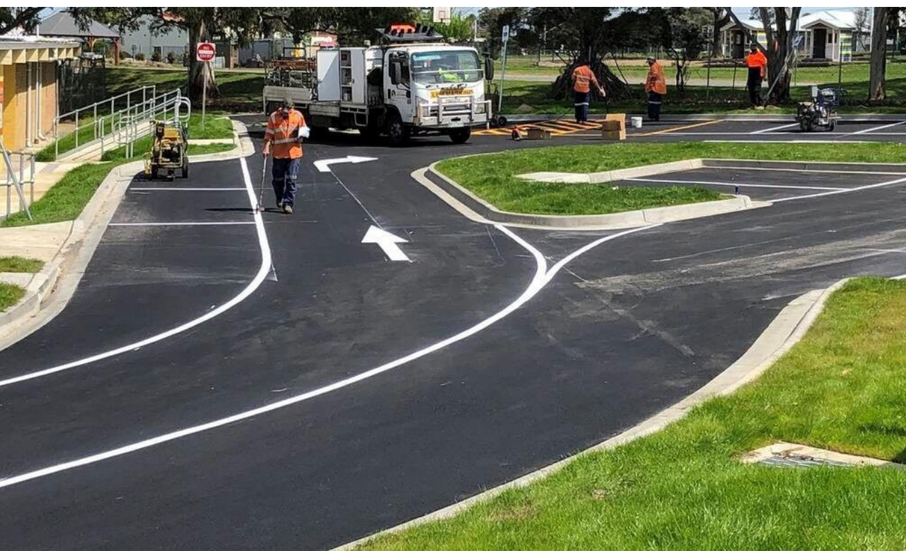
Council's Road Crew
