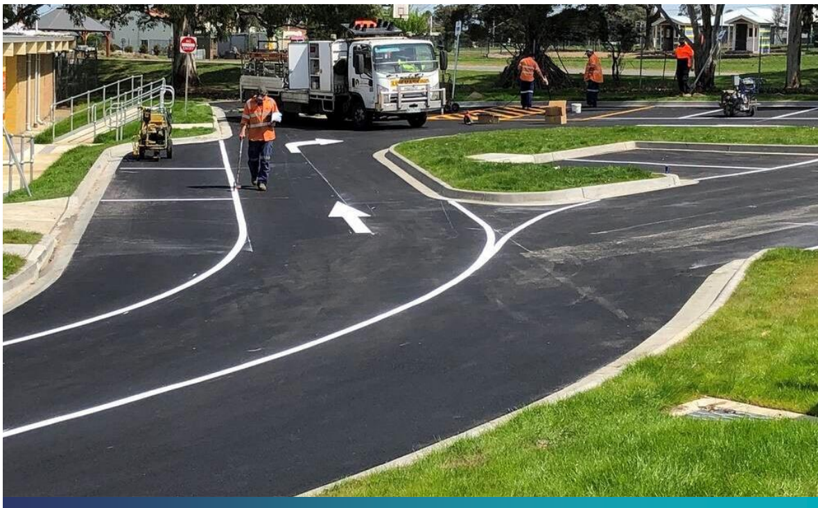
Council's Road Crew
