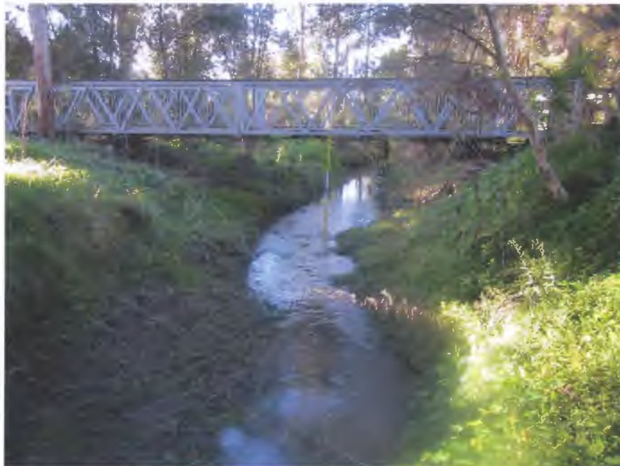
Appendix Figure A. 4 Pedestrian bridge adjacent to Foster Primary School – Stockyard Creek
