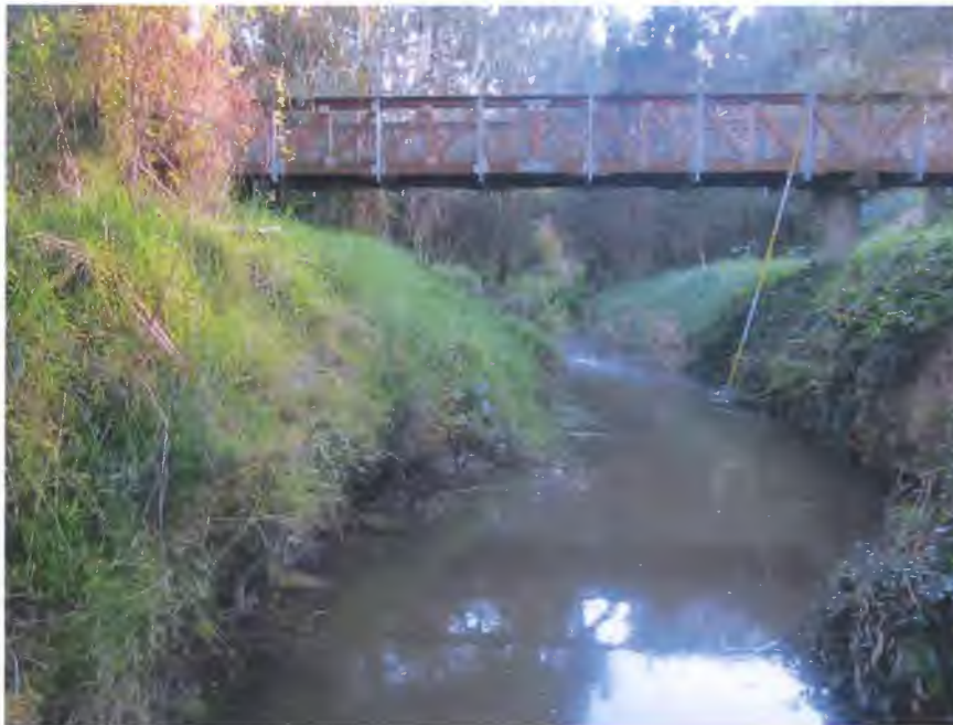
Appendix Figure A. 5 Pedestrian bridge adjacent to Scout Hall – Stockyard Creek
