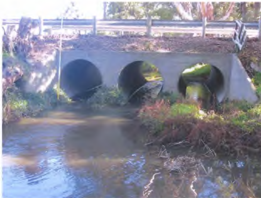
Appendix Figure A. 10 Elphicks Road culverts - Bennison Creek
