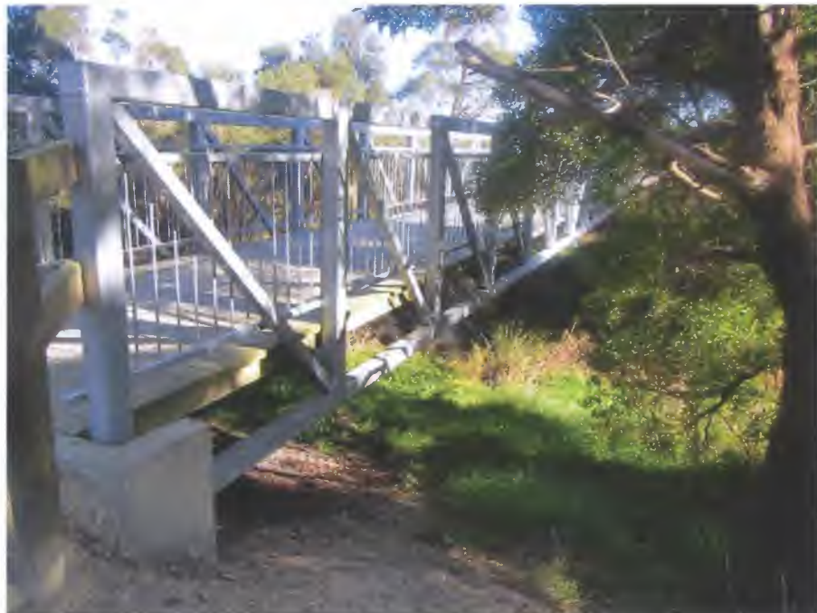
Appendix Figure B. 2 Rail Trail Bridge – Bennison Creek (2/2)
