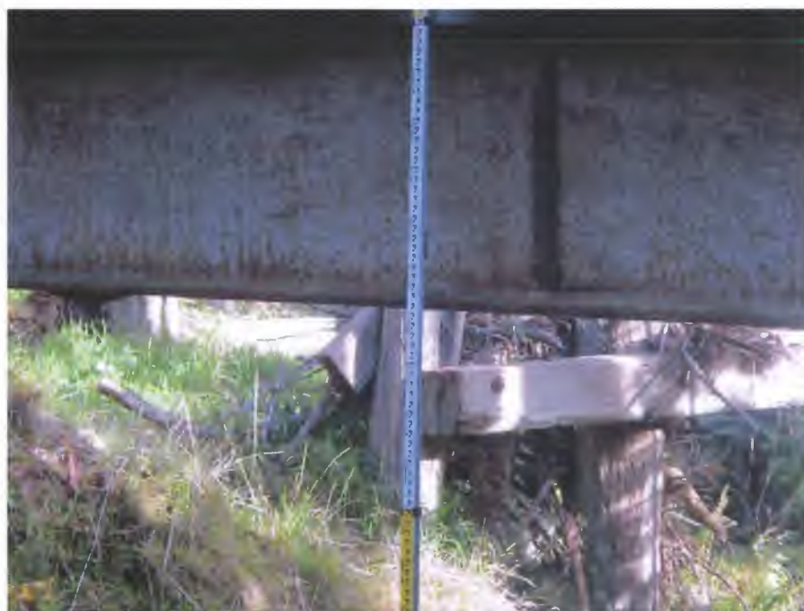
Appendix Figure B. 4 Rail Trail Bridge – Stockyard Creek (2/2)
