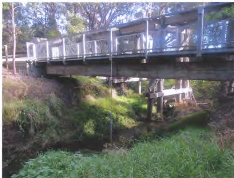
Appendix Figure B. 3 Rail Trail Bridge – Stockyard Creek (1/2)
