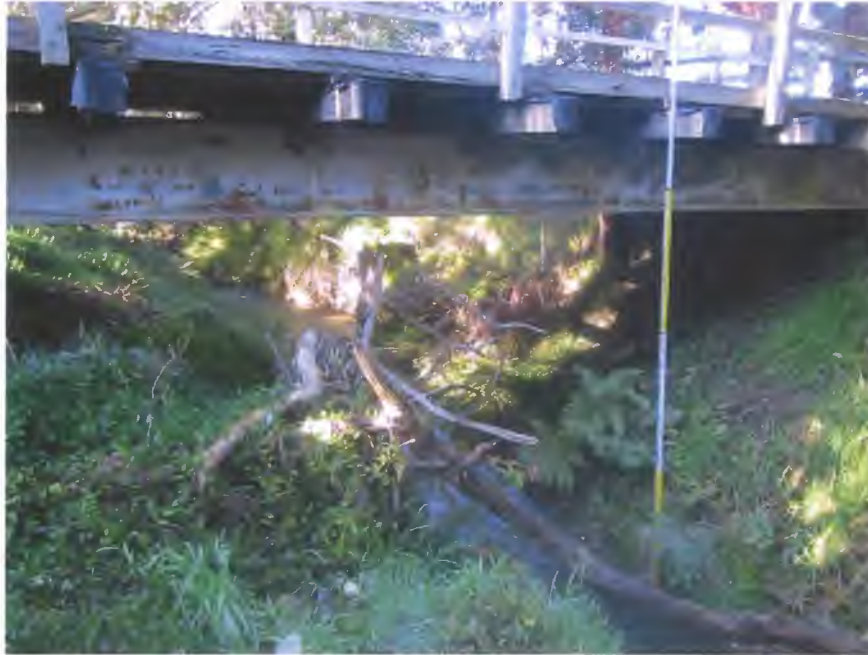
Appendix Figure A. 11 Jacksons Road bridge - Bennison Creek
