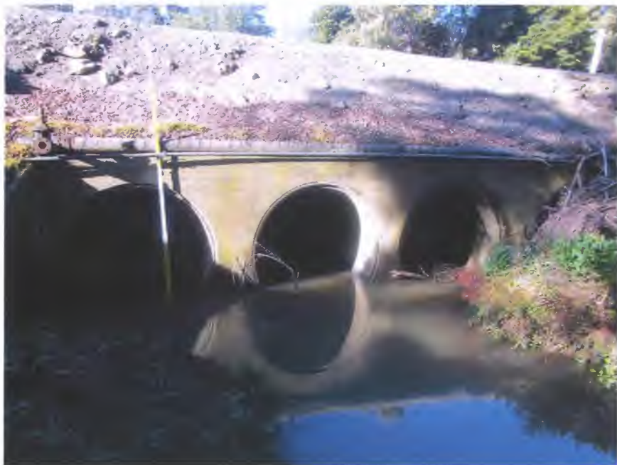
Appendix Figure A. 12 Ameys Track culverts - Bennison Creek
