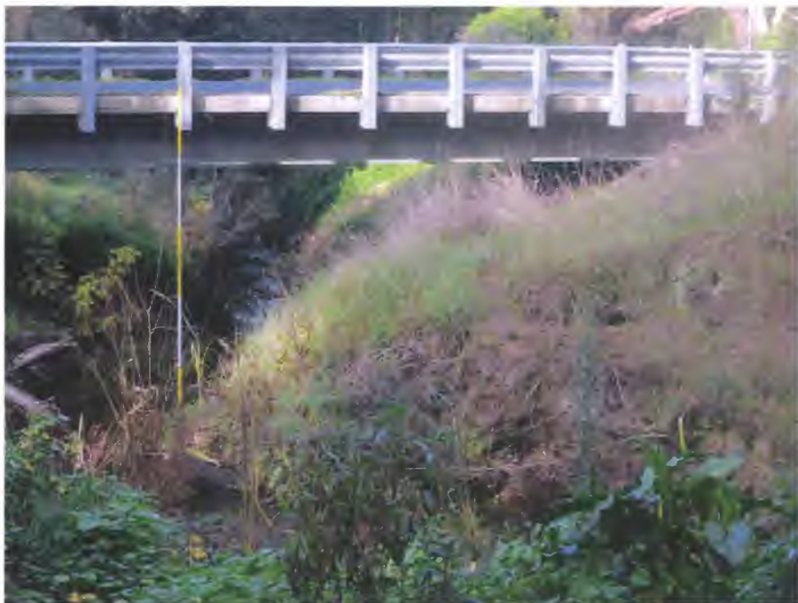
Appendix Figure A. 2 Dyrings Road Bridge 2 – Stockyard Creek (2/2)
