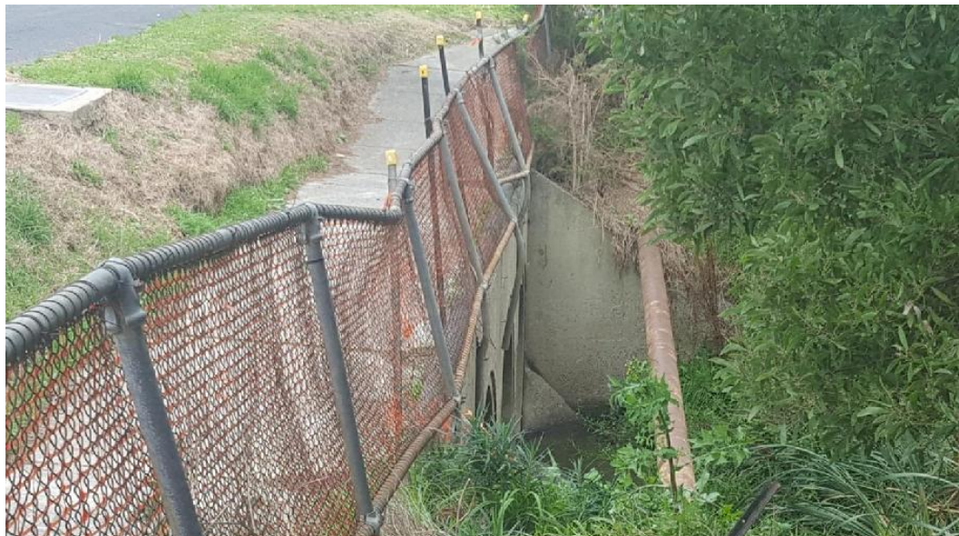
Figure 5.2 Upstream face of the Boundary Road culvert (09/04/2017)
