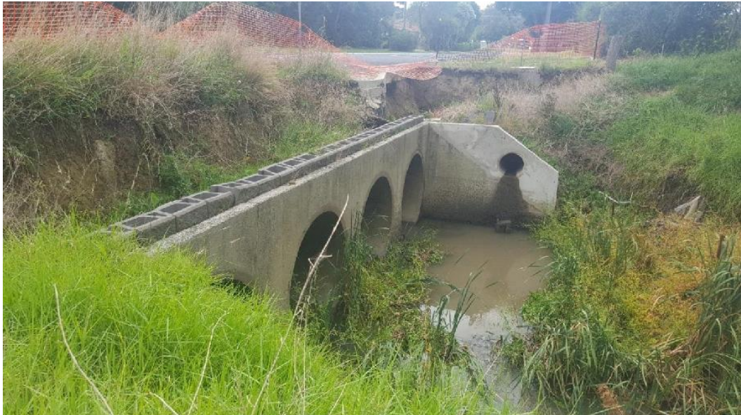
Figure 5.3 Downstream face of the Boundary Road culvert (09/04/2017)
