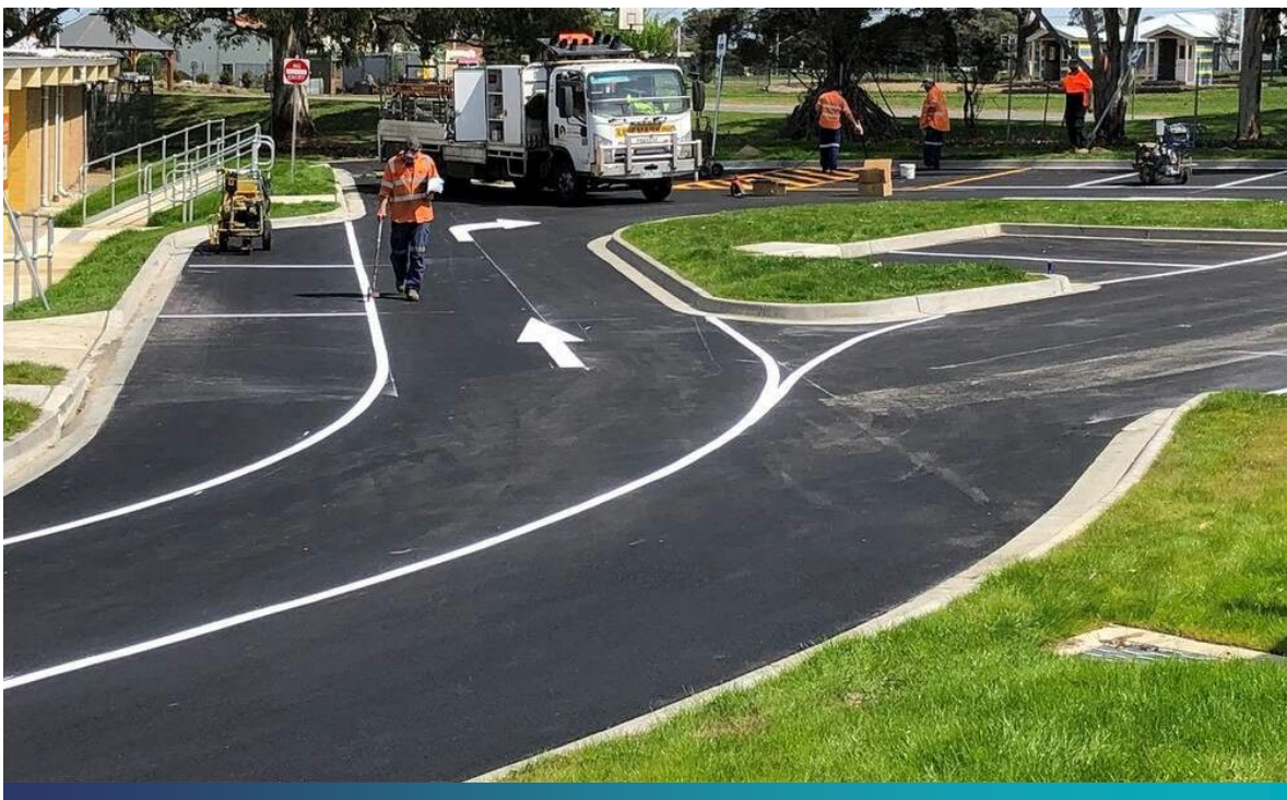
Council's Road Crew
