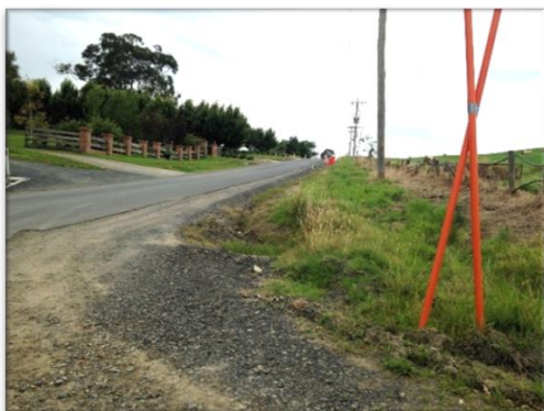
Figure 5.4: Available SISD looking east from Secondary Access Point
