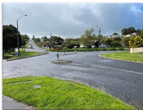
Figure 2.6: Bena Rd/ George St Intersection looking east towards Radovick St
