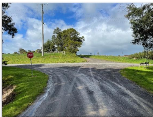
Figure 2.7: Bena Road/ Whitelaw Road Intersection, looking south
