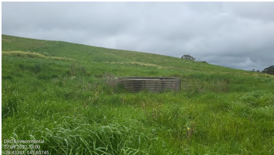
Plate 4: Concrete Water Tank present towards the north side, sealed off on top with one pipe connected to the water tank that runs into the ground
