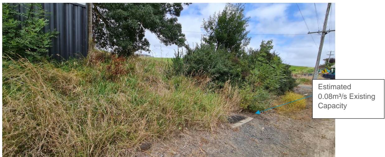
Figure 28. Existing Grated discharge at NE Corner
