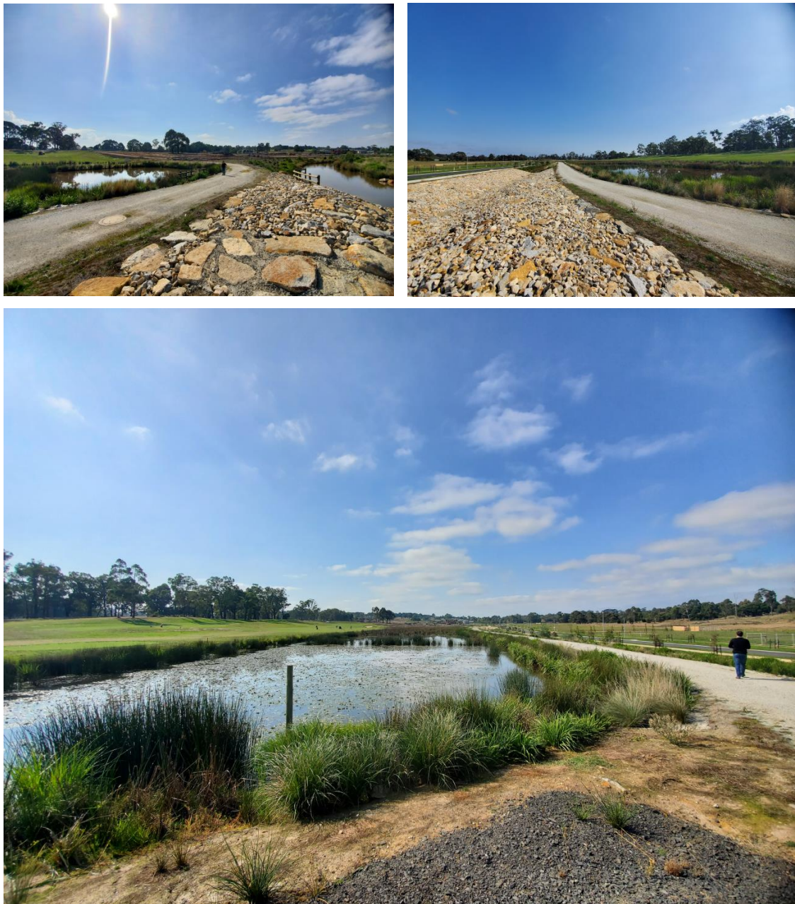
Figure 46. Drouin Wetland and Bypass Channel
