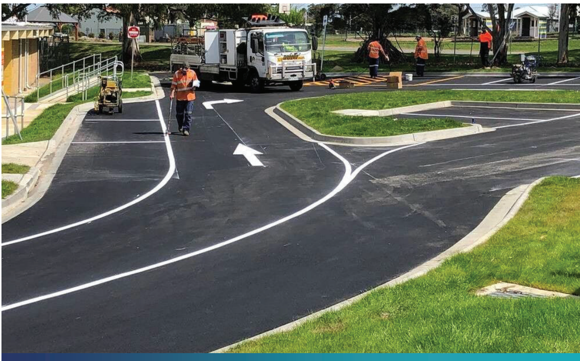
Council's Road Crew
