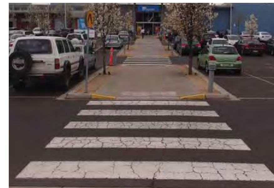
Example: central pedestrian refuge area to enable safe and comfortable pedestrian crossing
