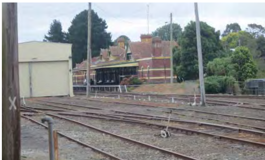
View of Railway Station from south-west of railway lines
