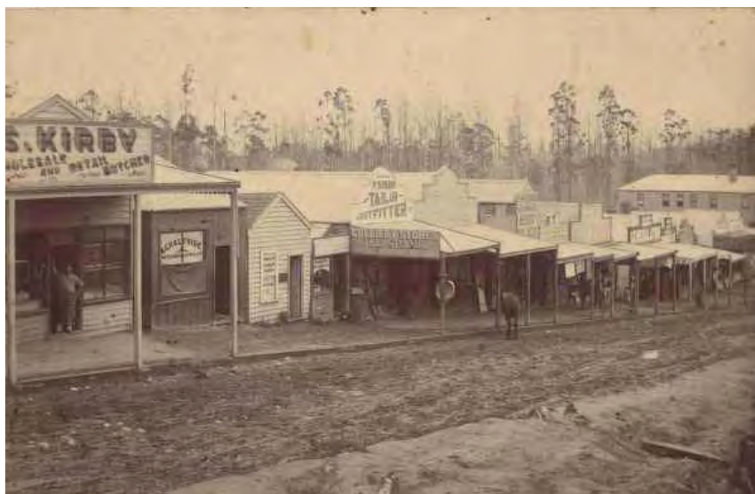
Historical photograph of Commercial Street
