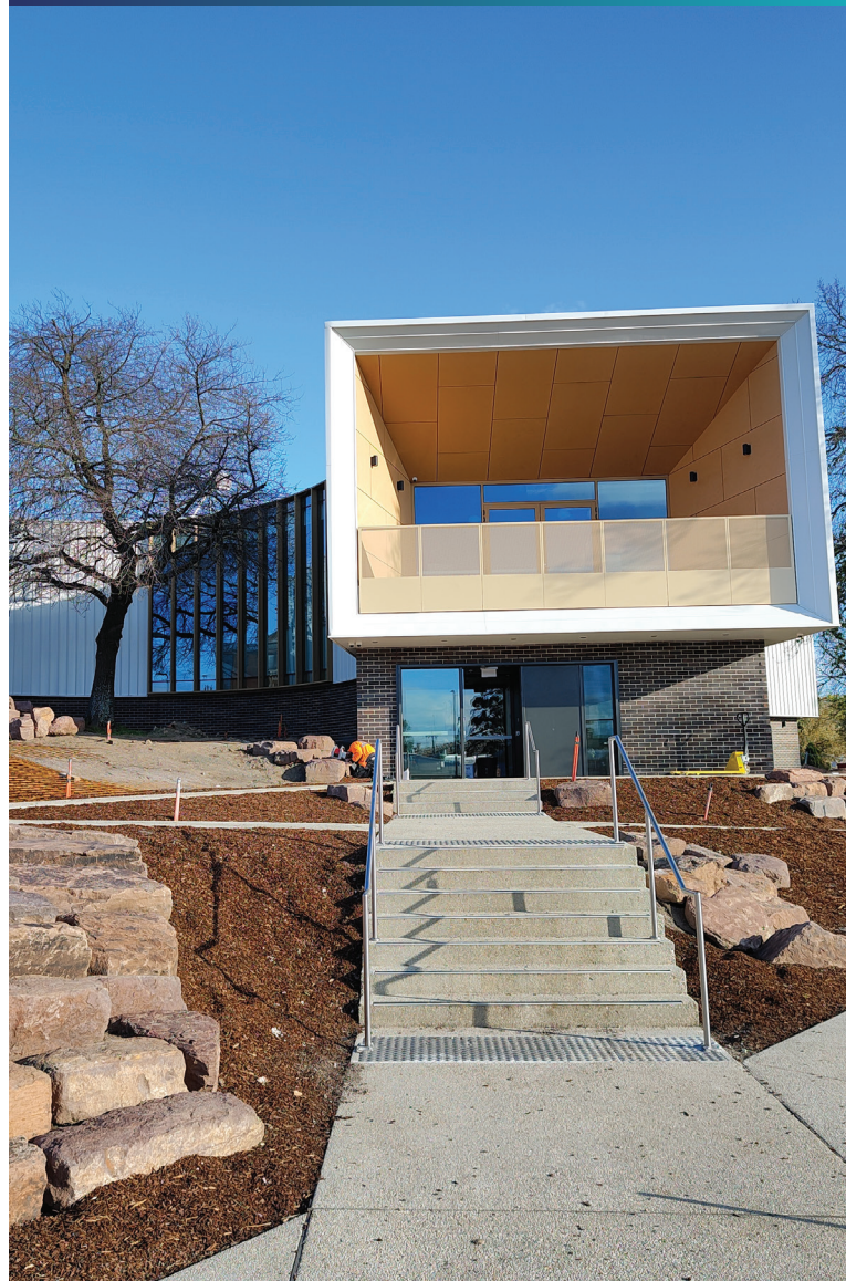
Pictured: The Korumburra Community Hub is close to completion
