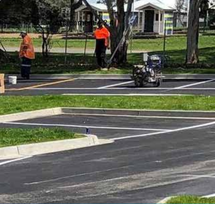
Road Works Crew
