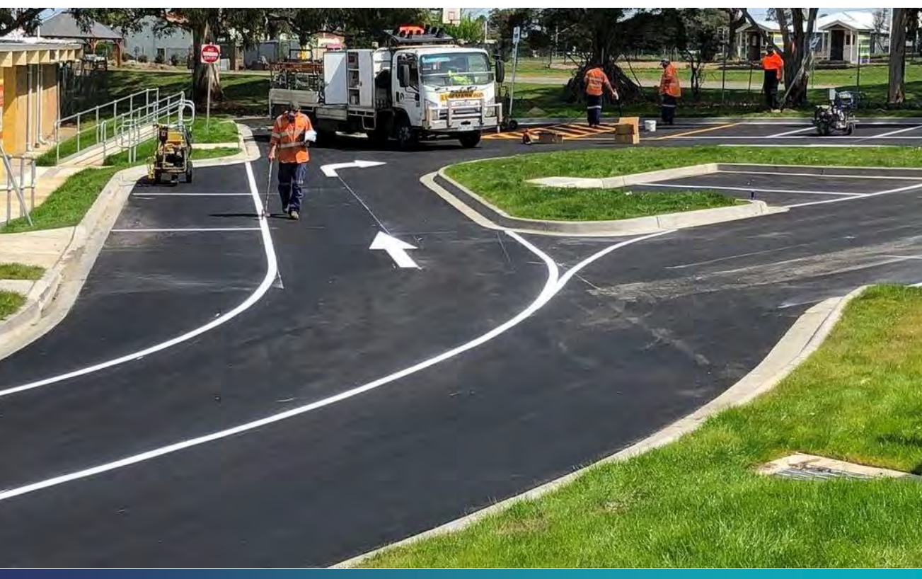
Council's Road Crew
