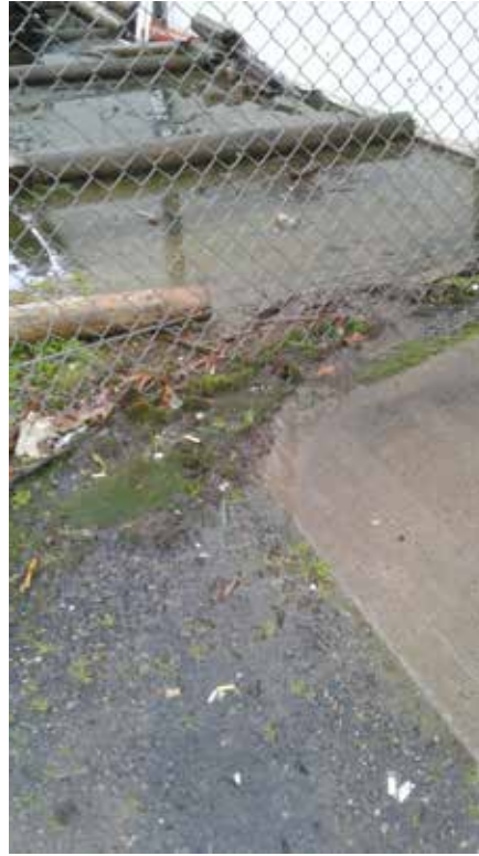
Walkway to the shops' entrances is particularly bad during wet weather. maintenance at 17 Ranceby Road which has caused many problems and safety hazards.
