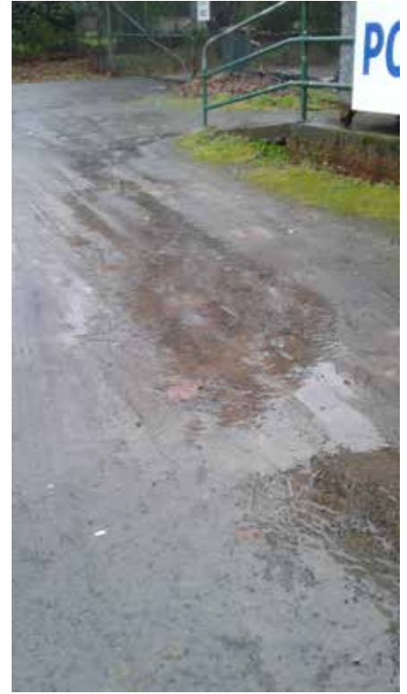
Spilling stormwater is clearly evident making its way across walkway and driveway sections.
