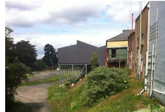
Western interface with private property
