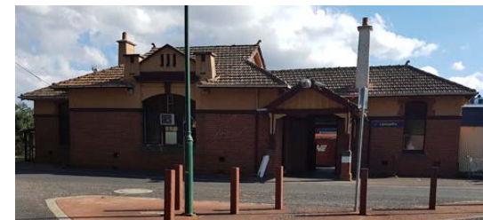
Main station building with waiting rooms
