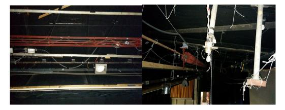
The stage grid is rudimentary with ad hoc rigging points for lighting bars, drapes and scenery. Bars are chained to the grid and are accessed by a moveable scaffolding tower from the stage.
