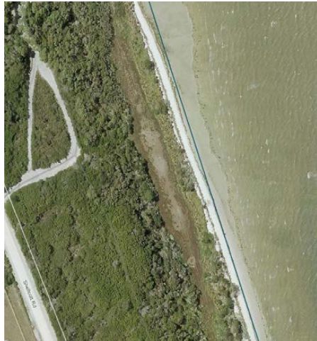
Aerial imagery of damage to vegetation from vehicle movements along the foreshore adjacent to Shellcot Road, Yanakie.
