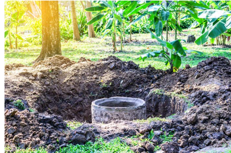
A wastewater system being installed
