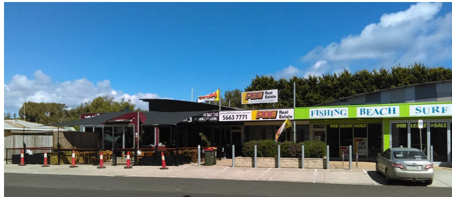
Temporary bollards provide pedestrian access at 144-116 Jupiter Bvd
