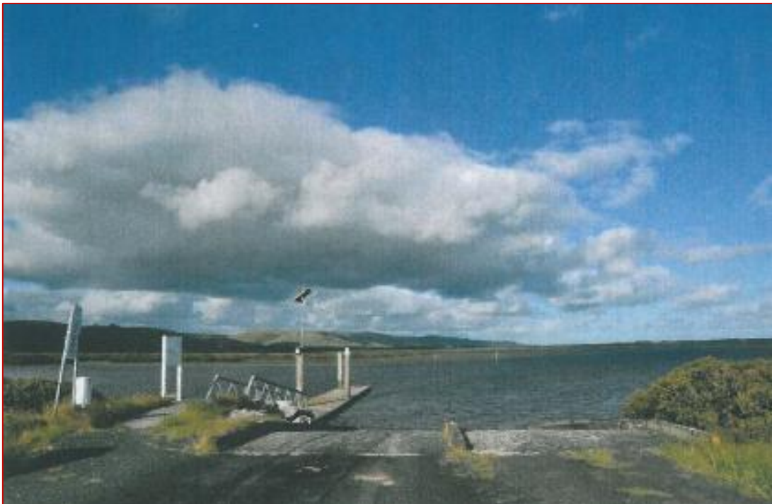
Figure 1.7: Toora Boat Ramp
