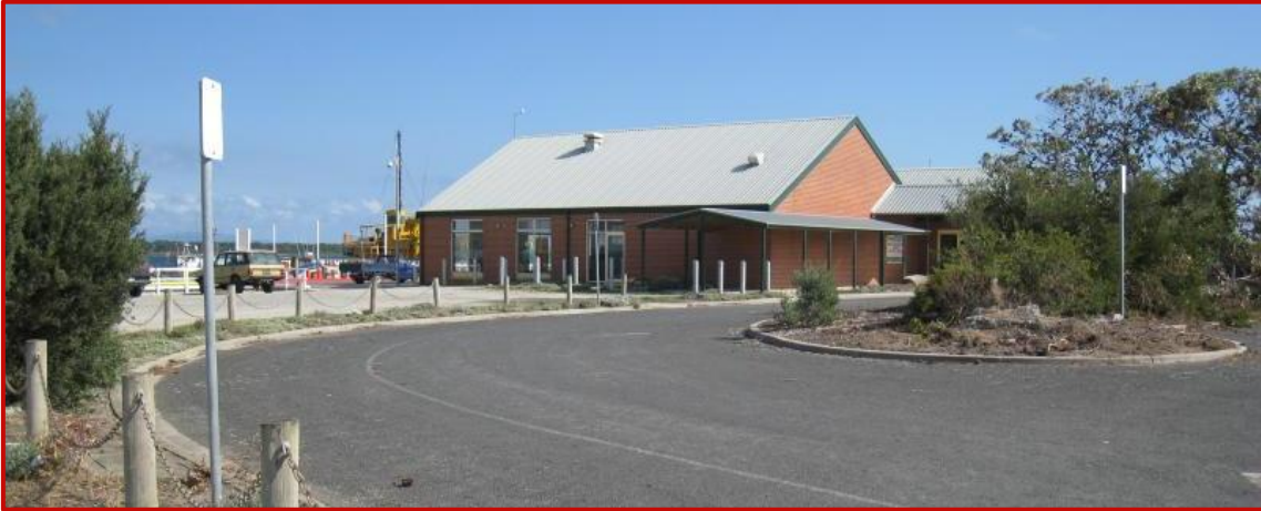
Figure 5.1: Port Welshpool Terminal Building
