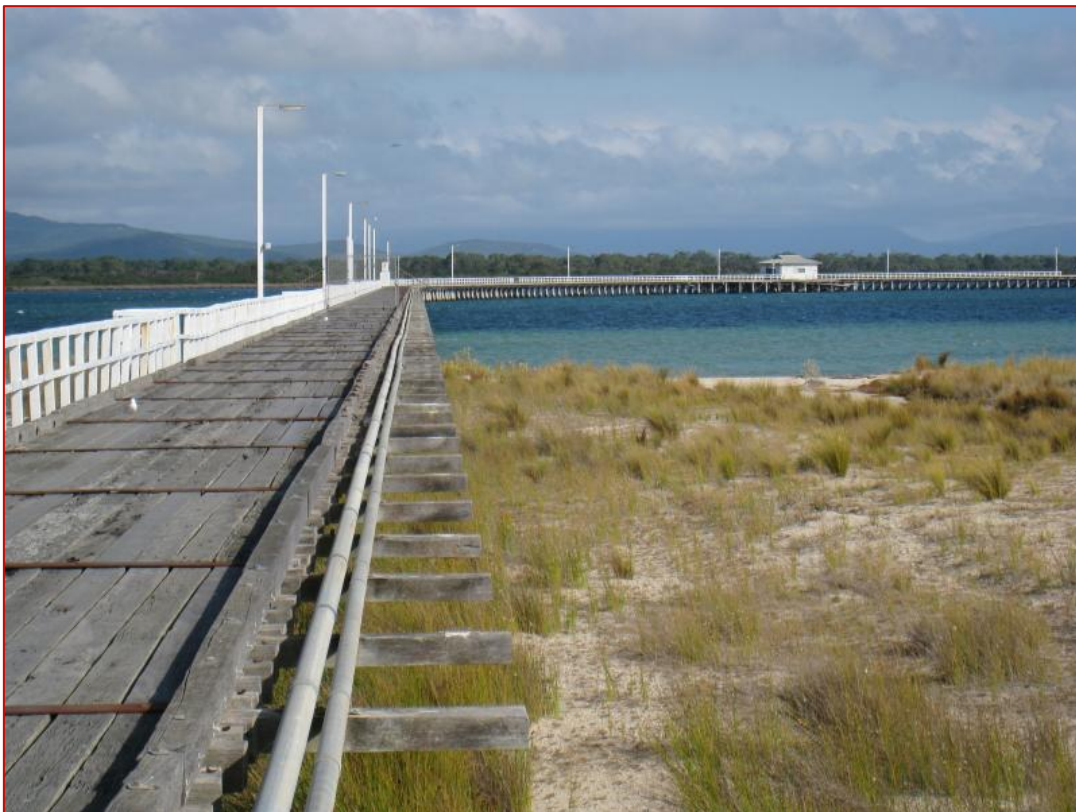
Figure 1.6: Port Welshpool Long Jetty
