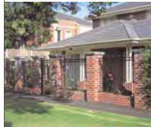
LEFT AND BELOW: ENSURE FRONT FENCES MAINTAIN GOOD VISIBILITY OF THE PUBLIC ENVIRONMENT AND PRIVATE ENTRANCES.
