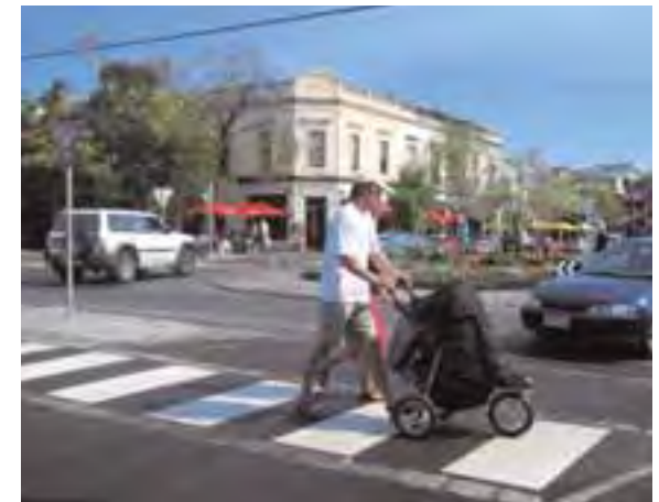
AS THE RADIUS OF THE KERB IS INCREASED, CARS ARE ABLE TO TRAVEL FASTER AND THE DISTANCE PEDESTRIANS HAVE TO CROSS INCREASES MAKING WALKING MORE HAZARDOUS. KEEP KERB RADII TO A MINIMUM AT INTERSECTIONS TO SLOW TRAFFIC AND PROVIDE THE SHORTEST POSSIBLE CROSSING DISTANCE FOR PEDESTRIANS AND OTHER USERS. ENSURE CROSSING POINTS ARE EASILY IDENTIFIED FOR ALL USERS.
