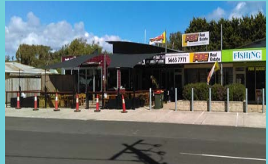
Temporary bollards provide pedestrian access at 144-116 Jupiter Bvd
