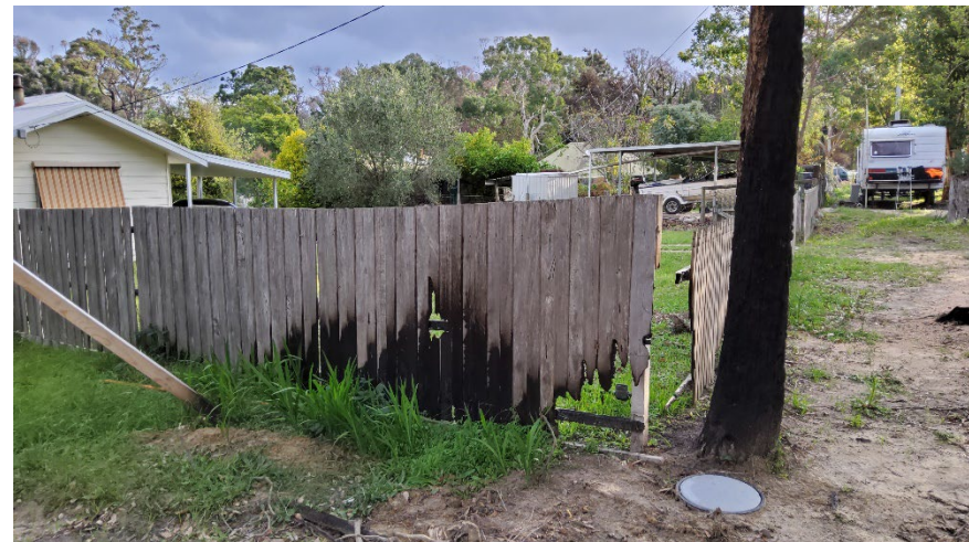
Figure 22: Example of the contribution of fencing to bushfire risk at a site level
