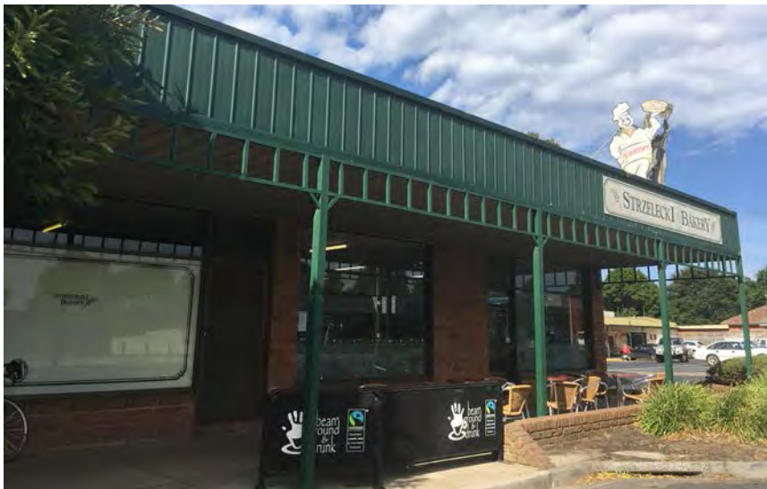
Shop front built to the boundary with verandah
