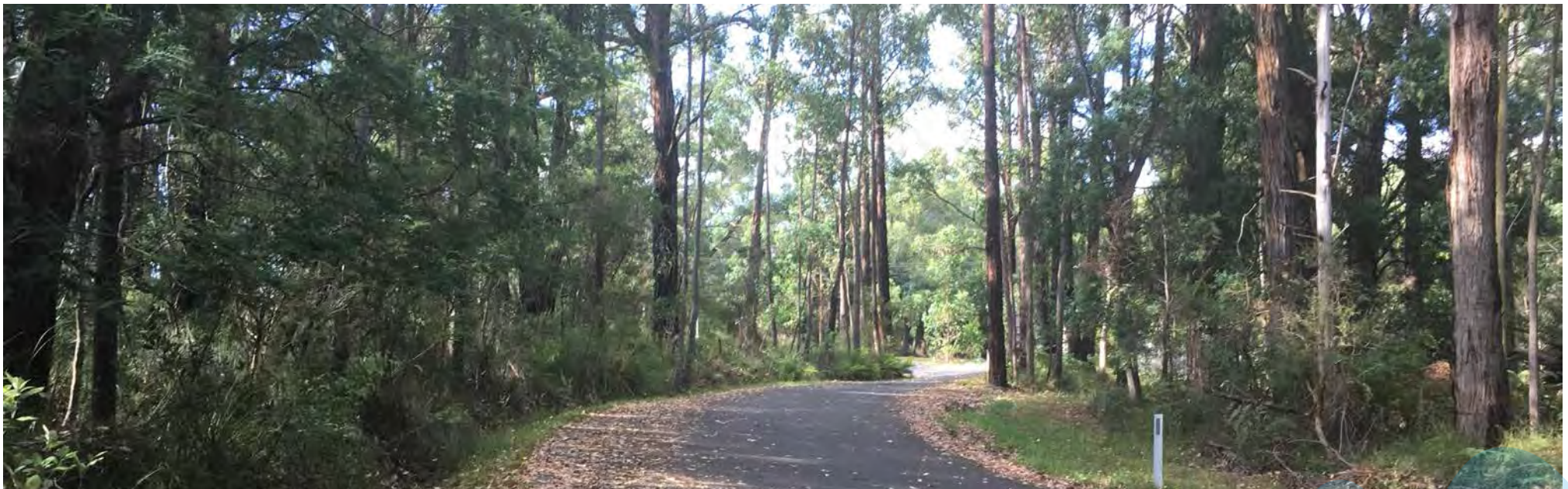
Jordan Way near Baths Road Reserve Ordinary Meeting of Council No. 412 - 24 May 2017
