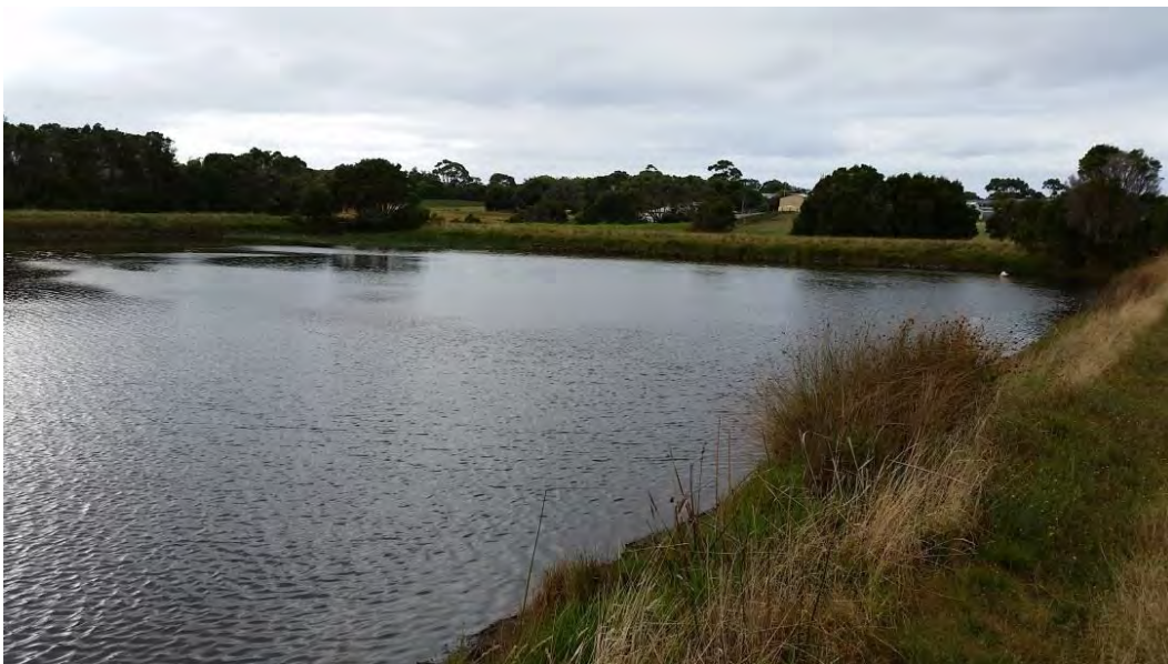
Figure 2 – Existing Walkerville Township Dam
